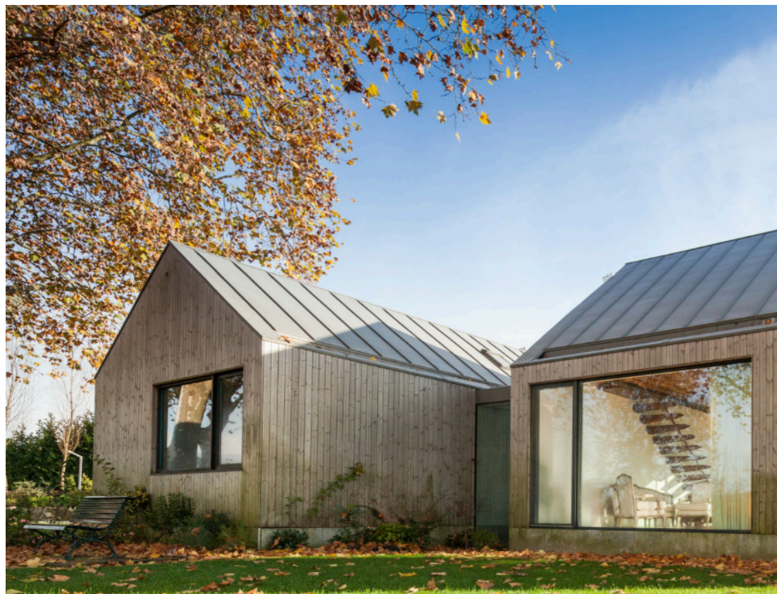
Timber precedent building with a standing seam zinc roof
