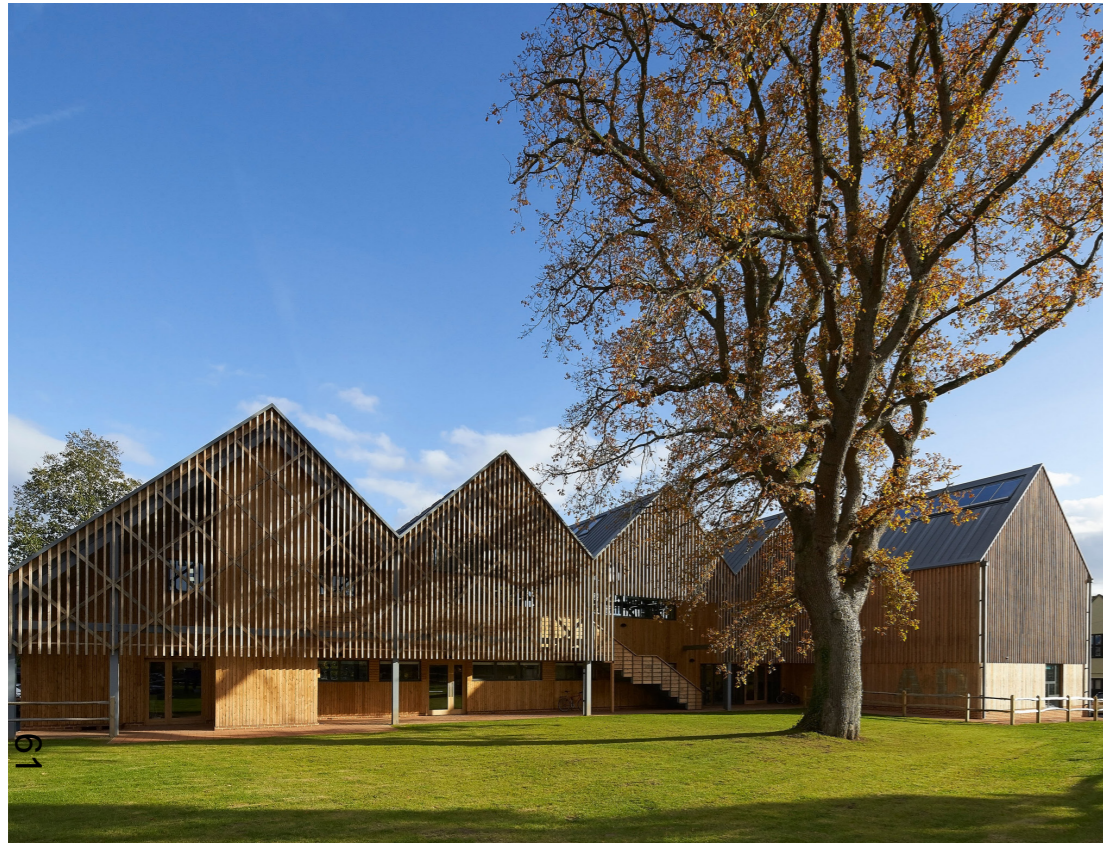
Timber precedent building
