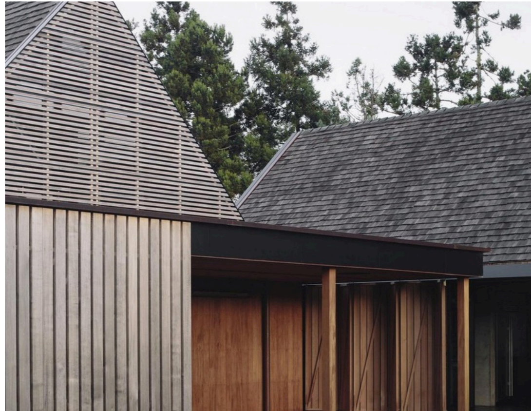
Timber precedent building
